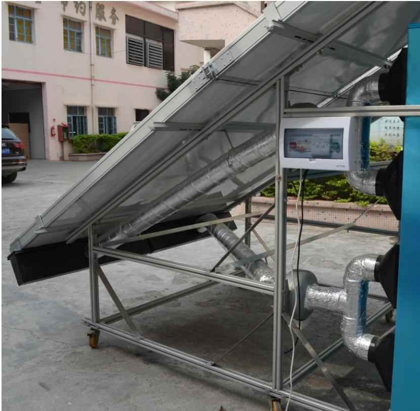
To maximize airflow efficiency, the Quad series draws air downwards through the solar air collectors to allow the hot air outlet ducts to be directed into cabinet. This can also be done either from a rooftop installation or from the ground outside a small building. The photo at left shows the manifolds, ducts and fans coming off the Quad collectors, and the control panel.
